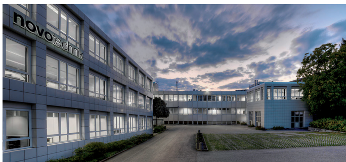
Headquarter Horbstrasse, Ostfildern (Germany)
