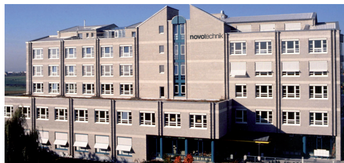
Production Brunnwiesenstrasse, Ostfildern (Germany)
